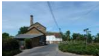
Overhead wires in vicinity of the mill
